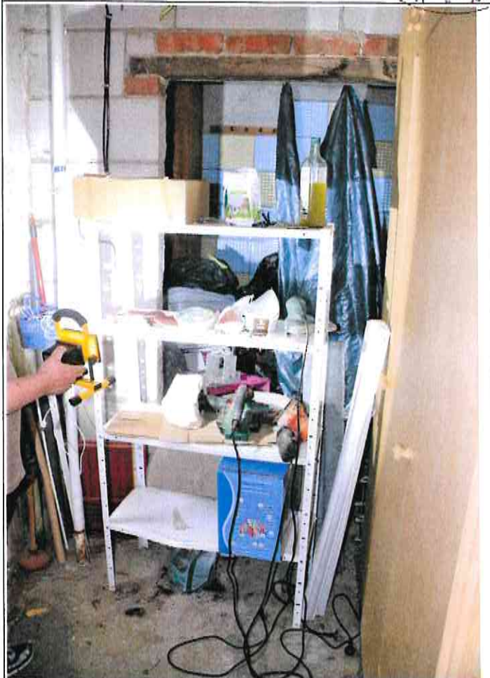
Erdgeschoss WE 1 Blick in Dusche
