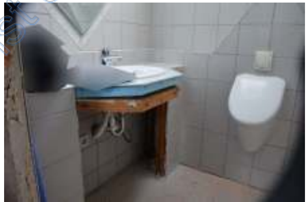
WC mezzanine Ebene
