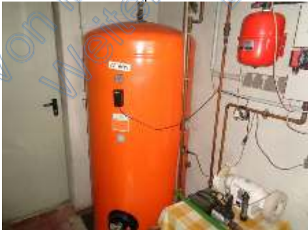
Warmwasser-Pufferspeicher
