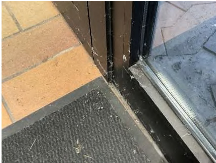
Schaufenster links Isoglas
