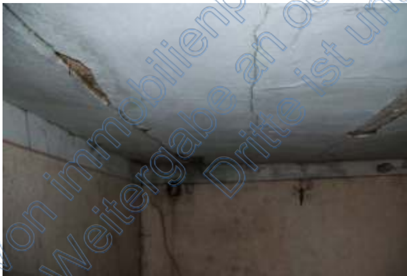
Detail Decke, massive Risses
