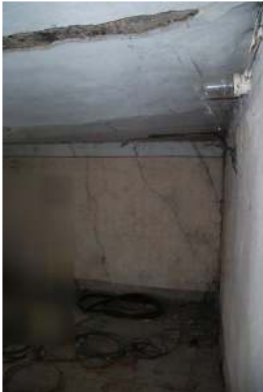
Detail massive Risses
