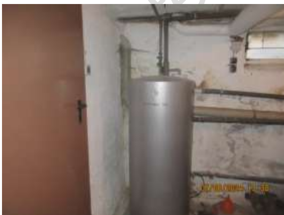
Warmwasserboiler
