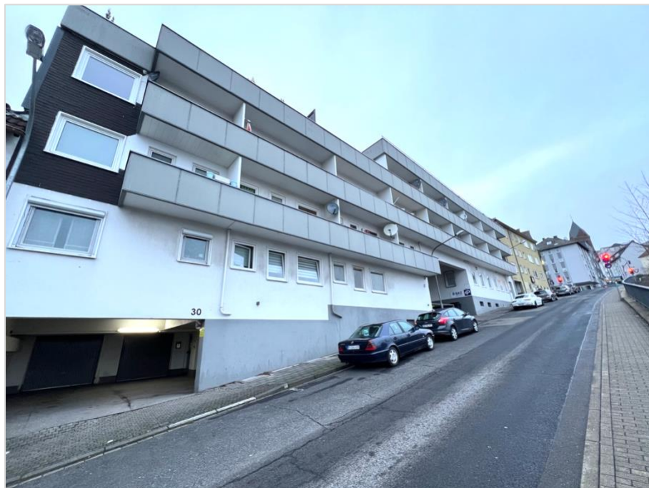
WET-Anlage Papenberger Str. 26, 28, 30
