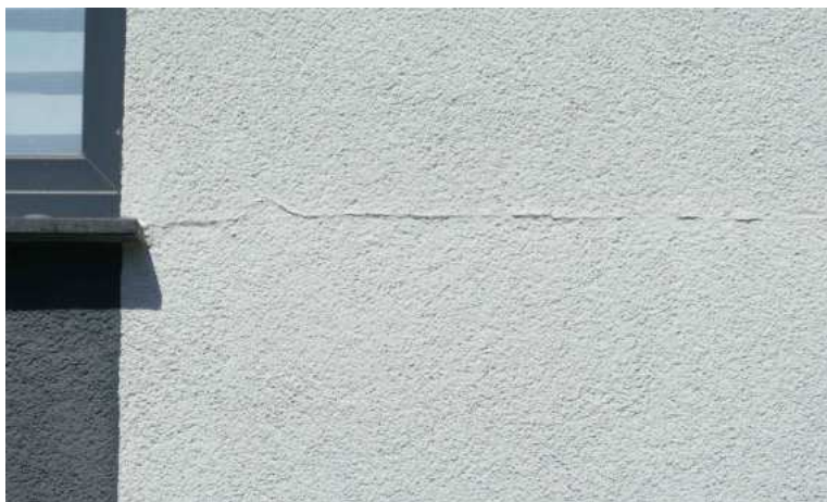
A1 Riss in der Fassade (WDVS)
