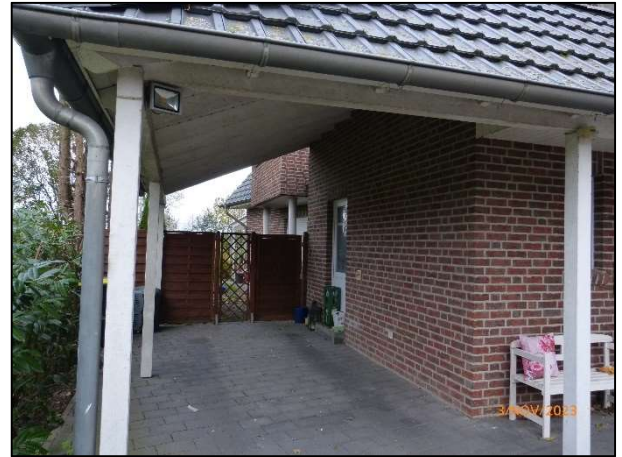
Blick in das Carport
