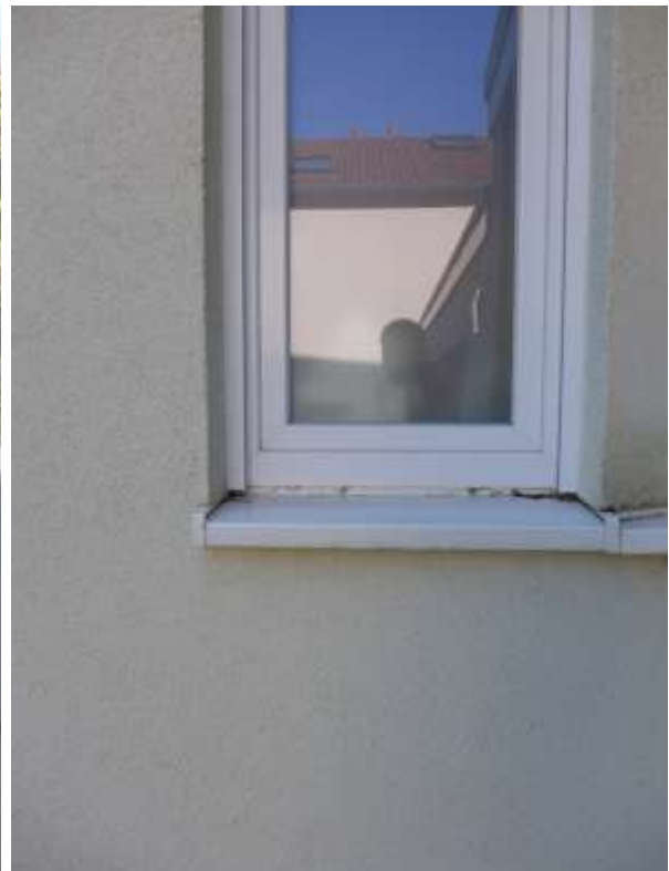
11 b Detail Fenster
