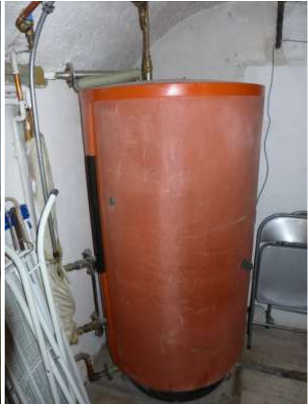
13 b Warmwasserboiler
