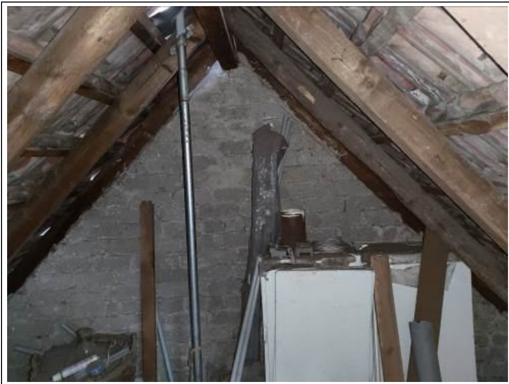
Blick in den Spitzboden
