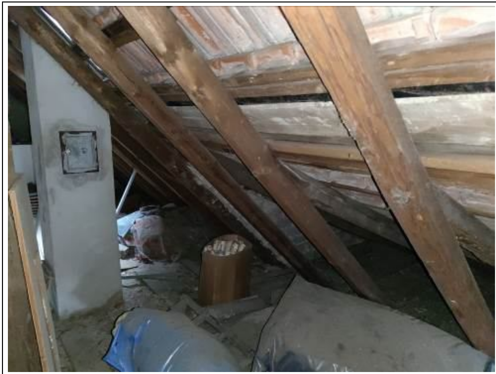
Blick in den Spitzboden
