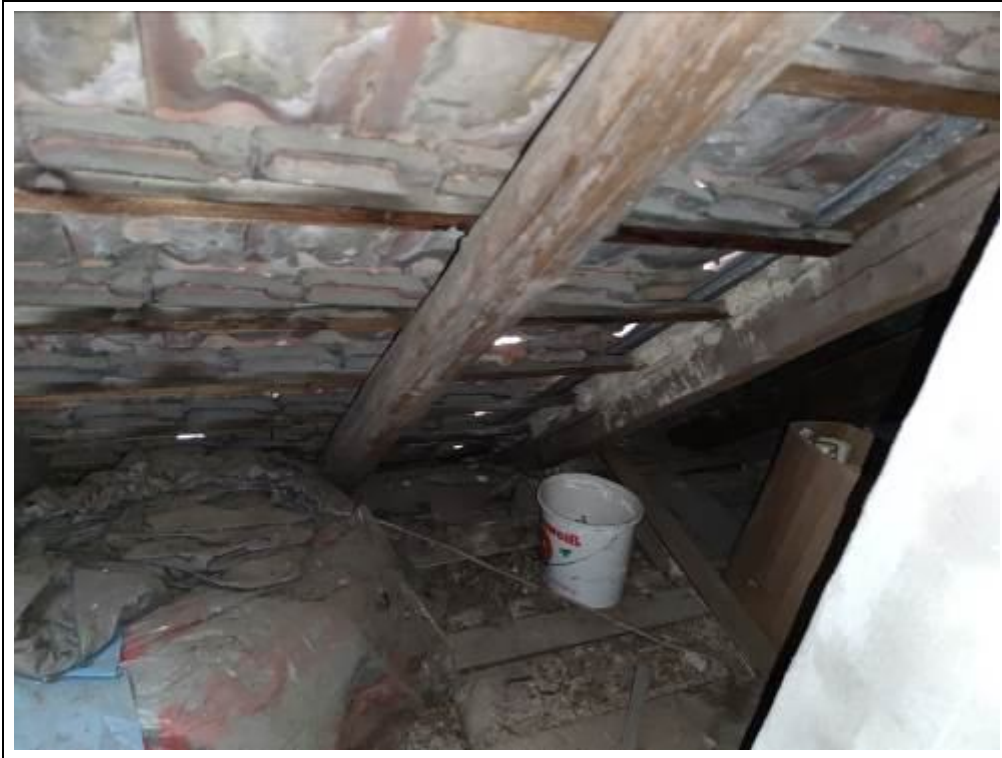
Blick in den Spitzboden
