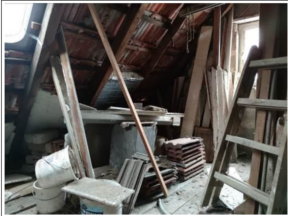
Blick in den Spitzboden
