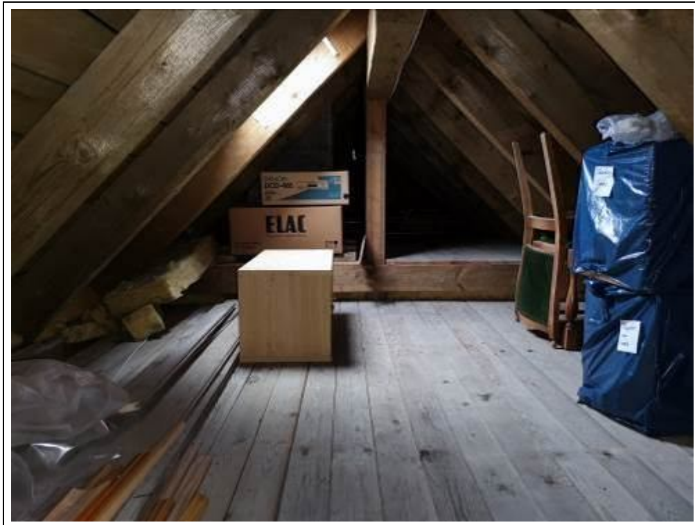
Blick in den Spitzboden
