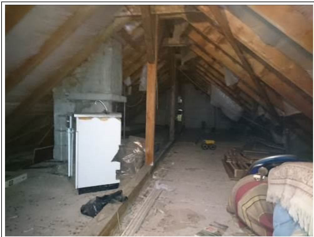
Blick in den Spitzboden
