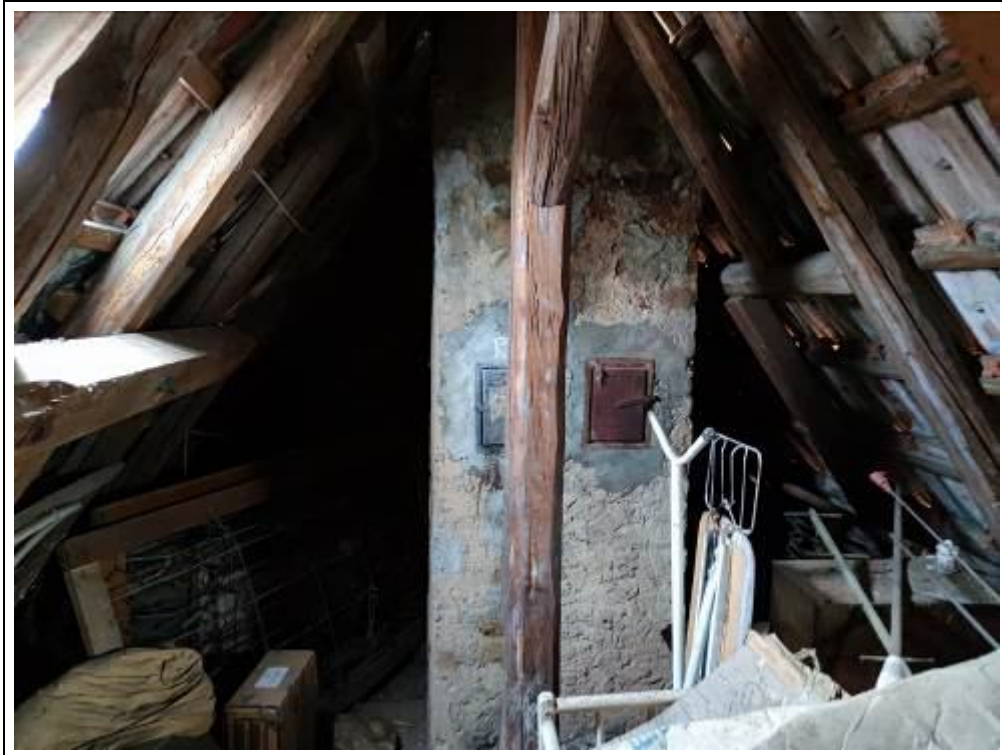
Blick in den Spitzboden
