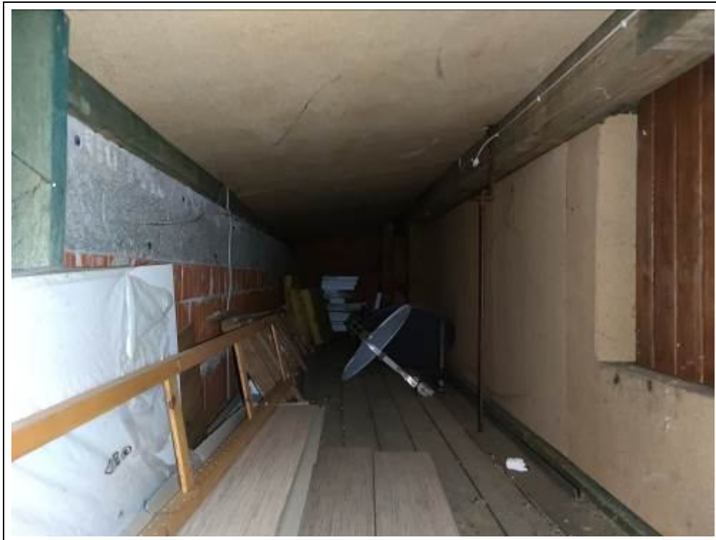
Blick in den Spitzboden
