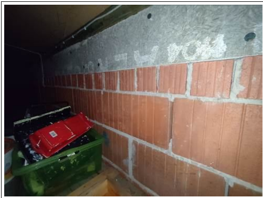
Blick in den Spitzboden
