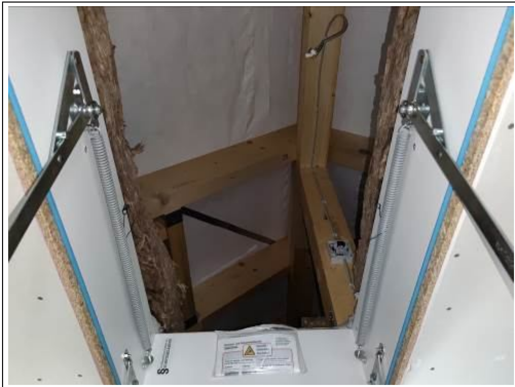
Blick in den Spitzboden
