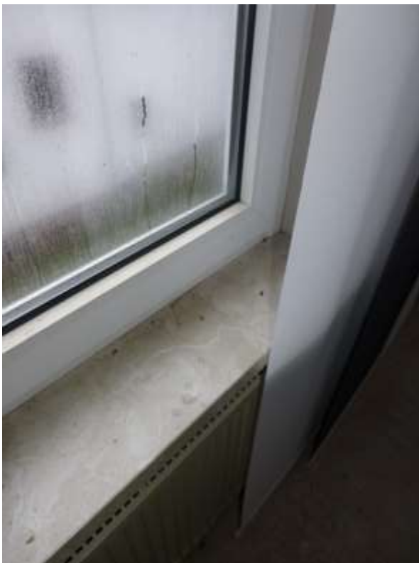
20 a Detail Fenster
