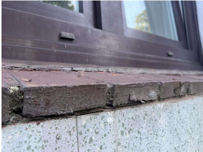
Detail Fenster/Fassade (WE Nr. 1)
