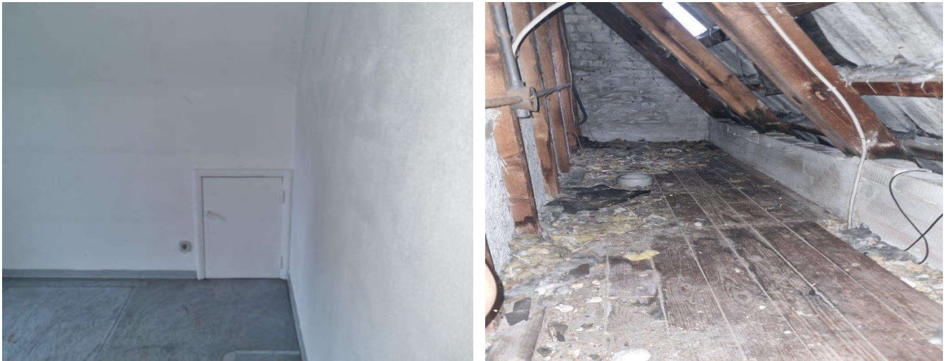
Blick in den Spitzboden
