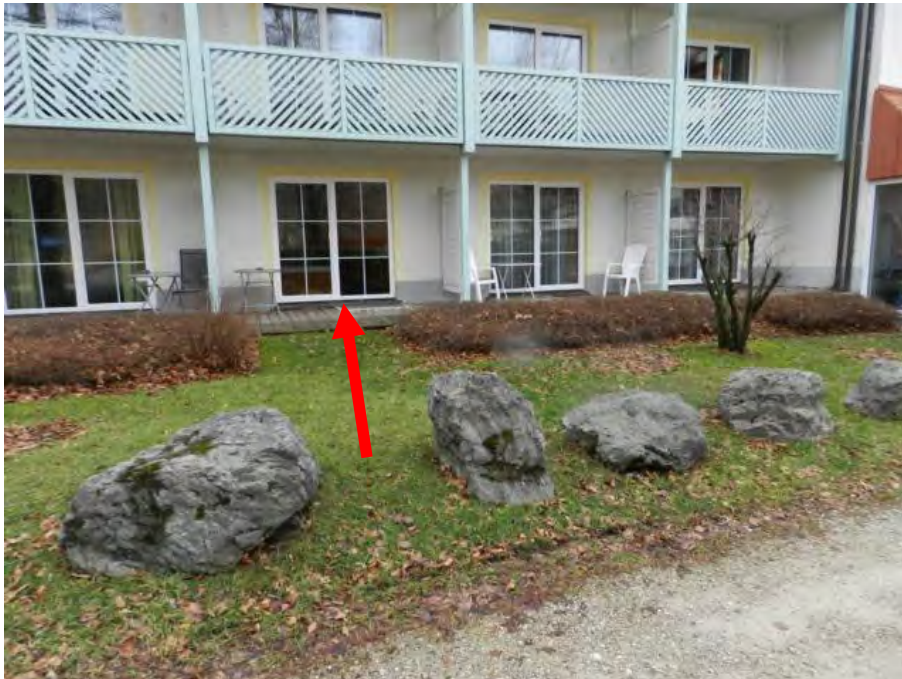
Apartment Nr. 3, Ostfassade
