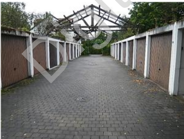
Garagenhof (Fl.Nr. 183/30) v. Norden
