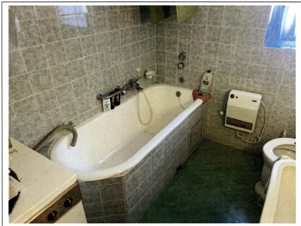
Foto 23: Blick in das Keller-Bad
