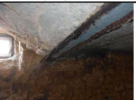
A photograph of a damaged vaulted ceiling in the basement, showing significant water damage and discoloration.                                     |
