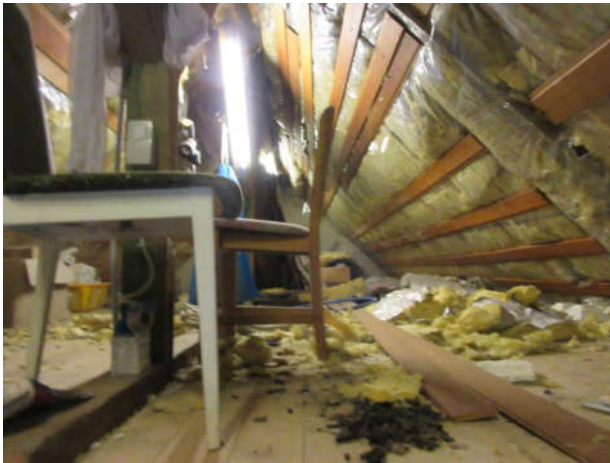
Blick in den Spitzboden
