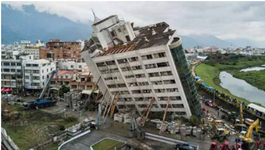
Figure 8.2 An earthquake devastated area
