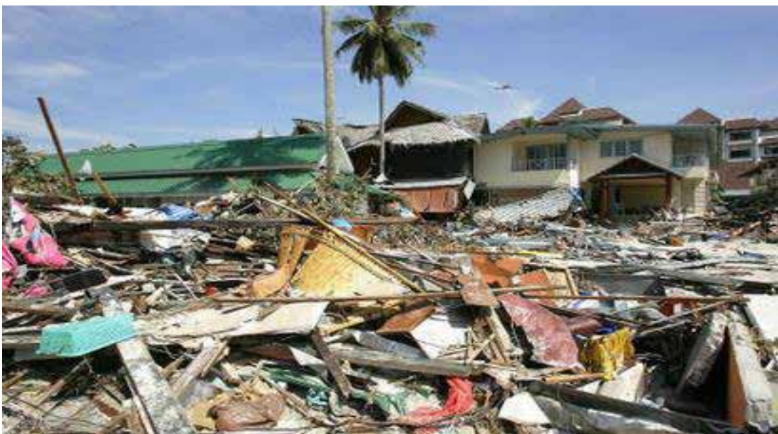
Figure 8.1 Infrastructure destroyed by Tsunami
