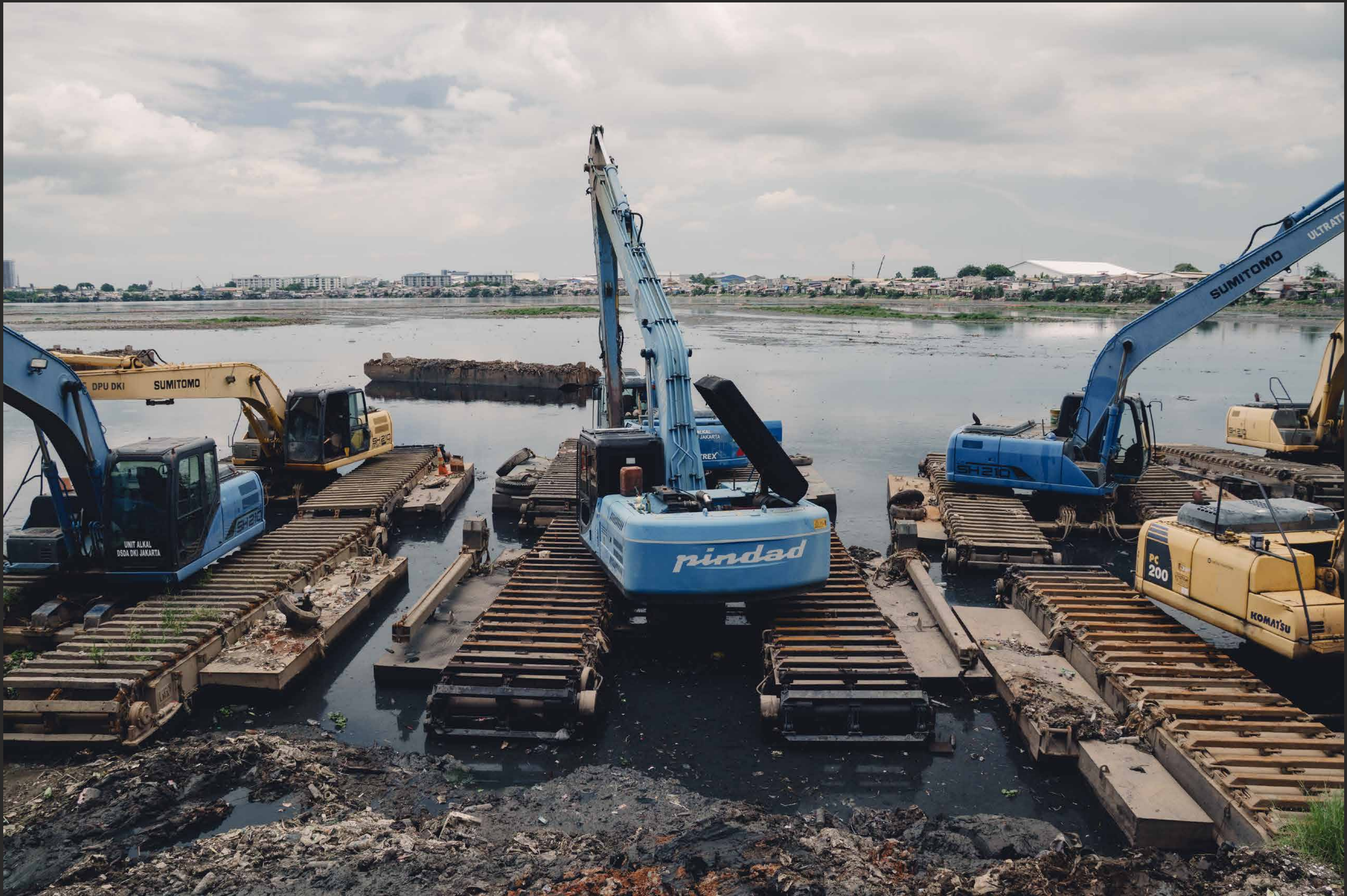
Amphibious excavators lined up along the coast for canal and river dredging.
