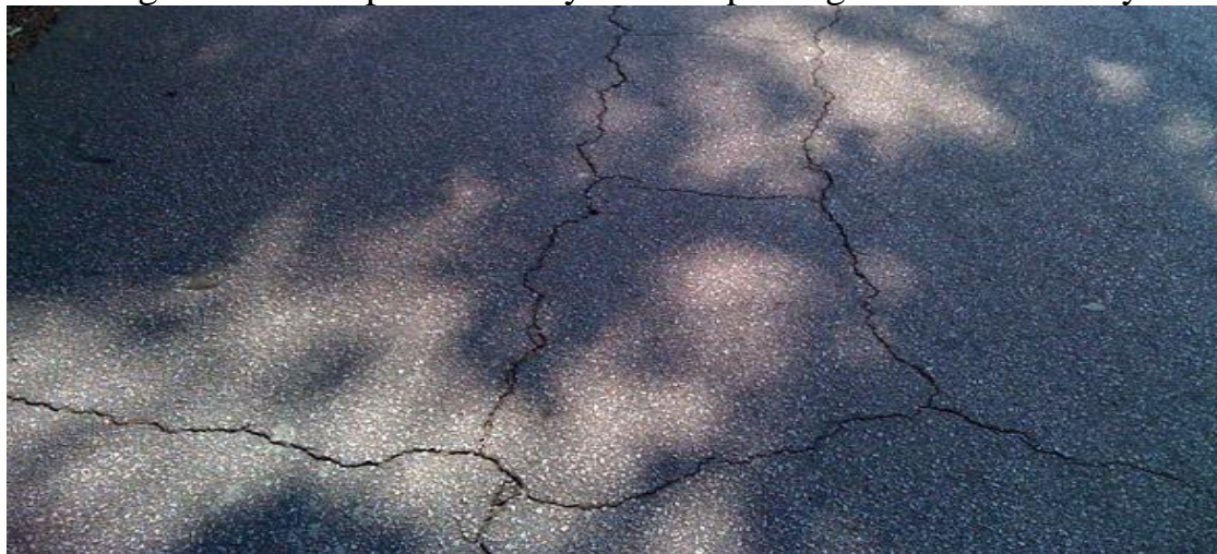
Fig. Block Cracking
