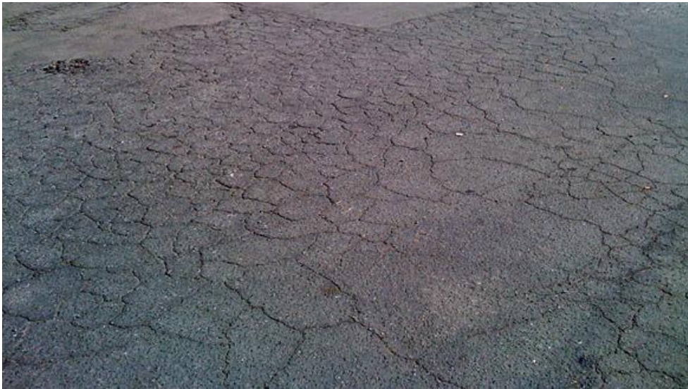
Fig. Alligator Cracking
