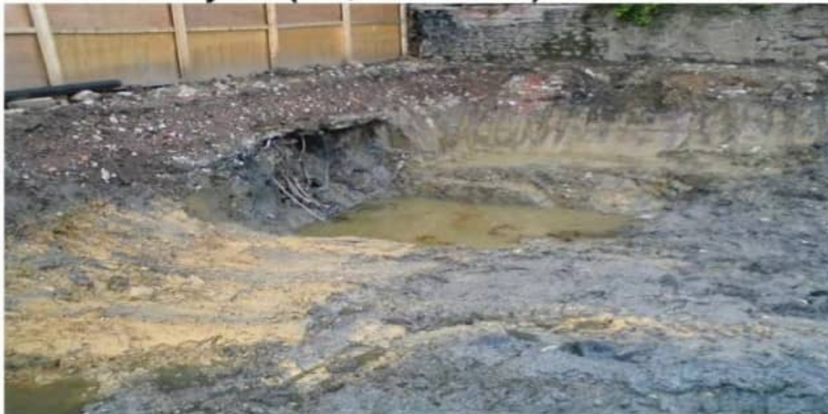
Excavation showing soil contamination at a disused gasworks
