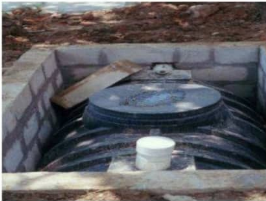
The septic tank partially installed in the ground
