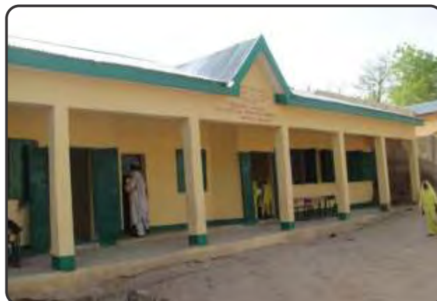
Plate 4.2: A block of classroom at Monguno LGA after intervention by Plan International in 2020
