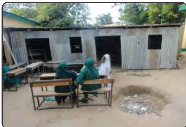
Plate 4.1: Temporary Classrooms Erected at Monguno LGA, before intervention by Plan International in 2019
