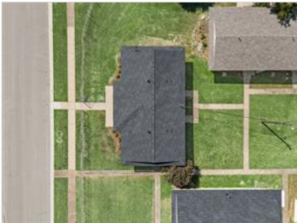
Aerial view; Architectural Shingle Roof
