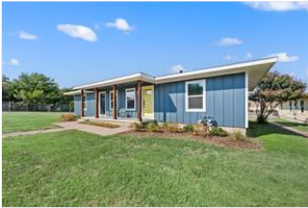
Board and Batten Fiber Cement Siding; Covered front rain porch
