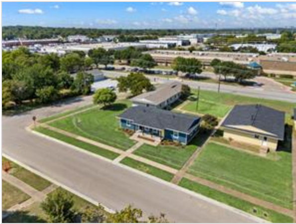
Aerial view; Architectural shingles
