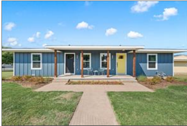
Fiber Cement board and batten siding; Covered front rain porch
