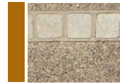
Exposed Aggregate Concrete with Granite Sett Band
