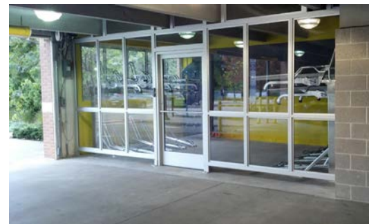
Completed parking garage retrofit
