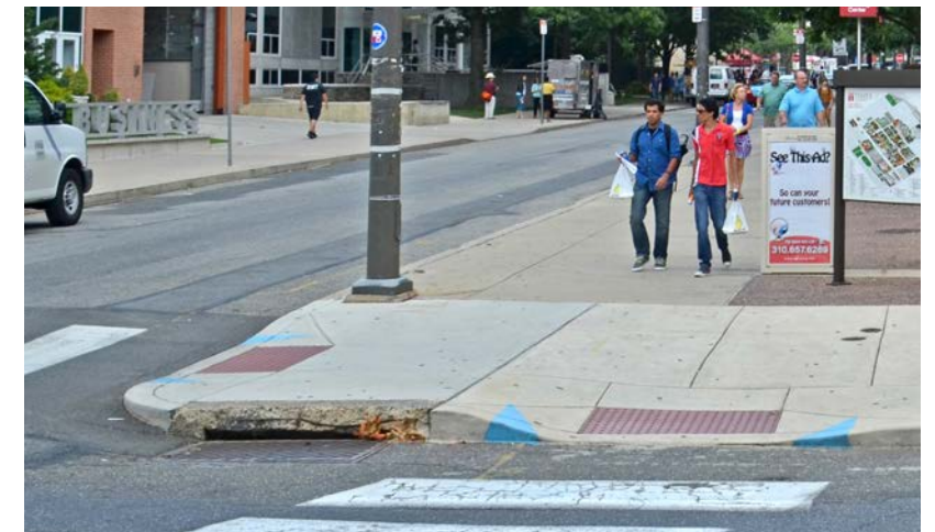
City owned combined storm and sanitary sewer
