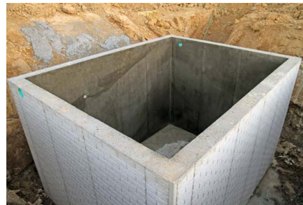
Underground concrete cistern
