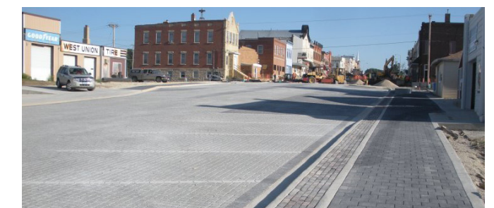
Parking lot using porous unit pavers
