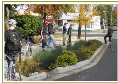
Curb extension with bioretention
