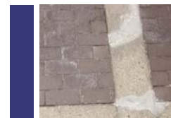
Brown Brick with Concrete Band
