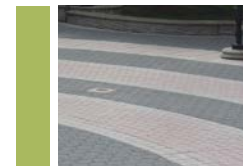
Black Hex Asphalt Pavers with Concrete Pavers
