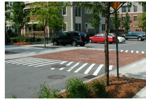
Example: Traffic calming features (raised crosswalk) in the neighborhoods surrounding Harvard and MIT in Cambridge, MA.
