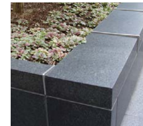
SkateStoppers® metal inserts at joints
