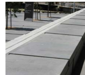
SkateStoppers® metal inserts at joints
