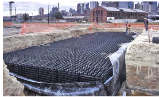
Raintank system being installed
