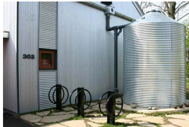
Metal rain barrel type cistern
