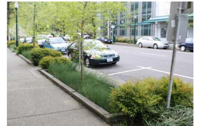
Unpaved stormwater tree trench
