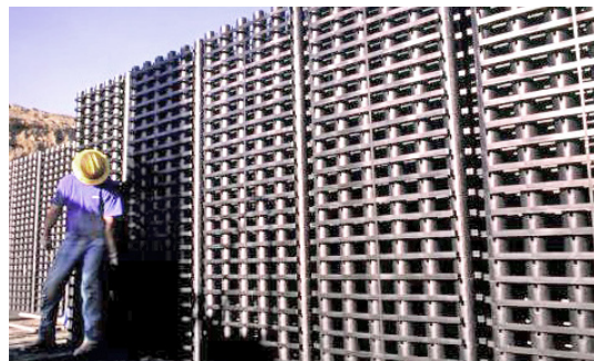
Raintank system stacked for installation
