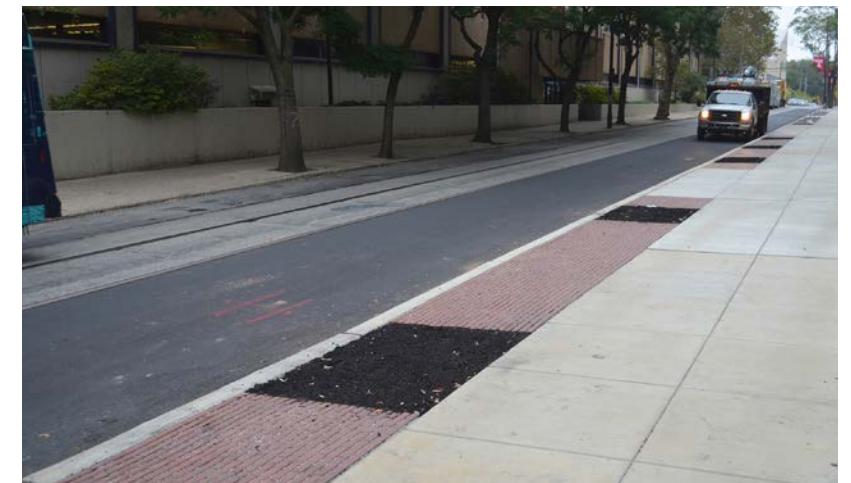
Examples of GSI: Newly installed tree trenches on Temple's campus
