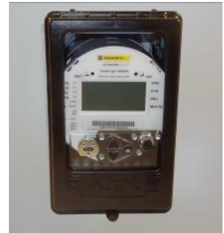
ION 8650 Retrofitted into Westinghouse/ABB cutout
