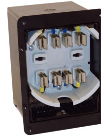
3. Retrofit Panel Adapter Installed
