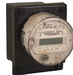
4. Installed with Aclara kV & cover
