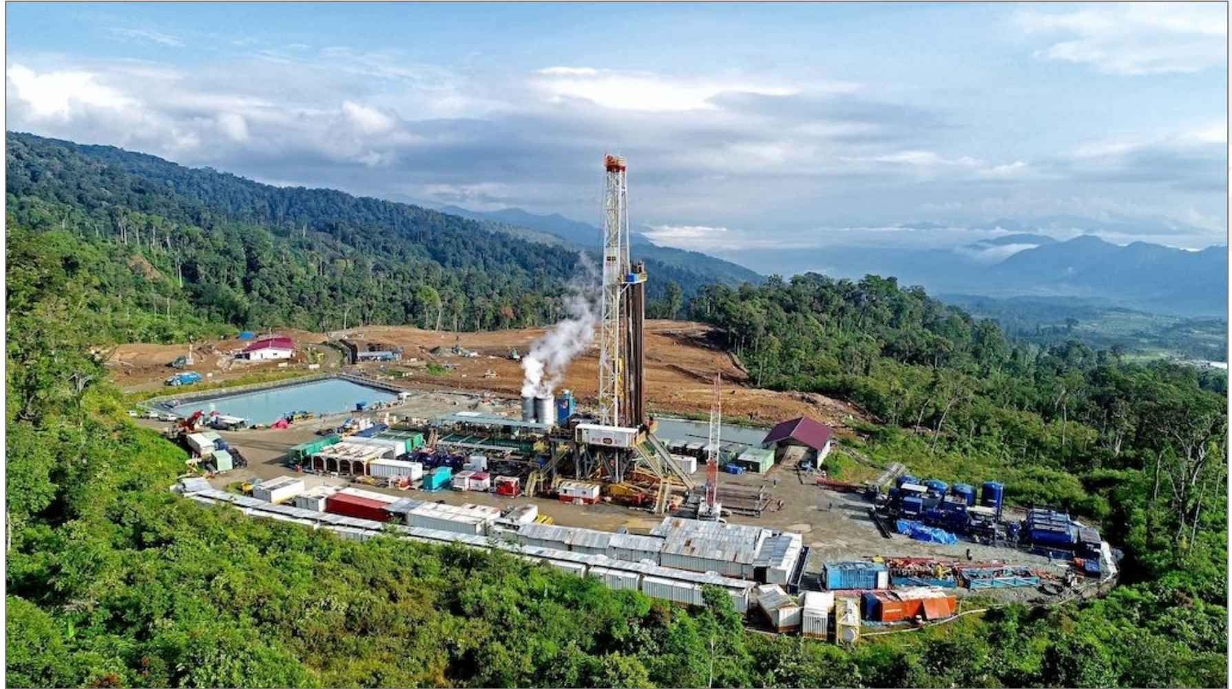
Muara Laboh Geothermal Field, Sumatera, Indonesia Source: Sumitomo Corp, retrieved from Thinkgeoenergy
