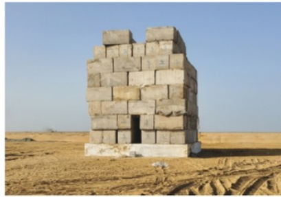
Concrete loading blocks placed on top of test footing
