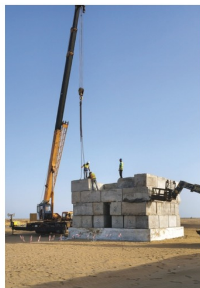
Concrete loading blocks applied to footing
