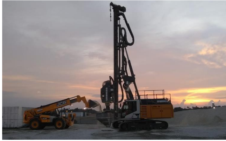
Fig. 3. a) Construction Method of the Rammed Aggregate Pier System and b) photograph of RAP installation at the site
