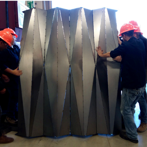
Fig. 7 Students in Flat Force Fold Form research studio preparing to move a 360lb roof piece prior to installation.
