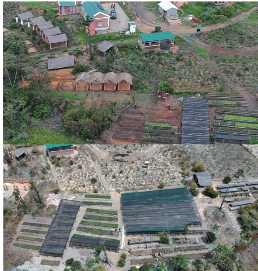
Upper photo – Drone view of the Vahatra infrastructure at Ambohitantely, the biological station buildings to the left of park vehicles, behind to the left the new sanitary facilities, and slightly below tent lean-to structures; in the lower section the tree nursery. Lower photo – A close up of the tree nursery with a good portion of the beds covered with a sun-protecting mesh.
