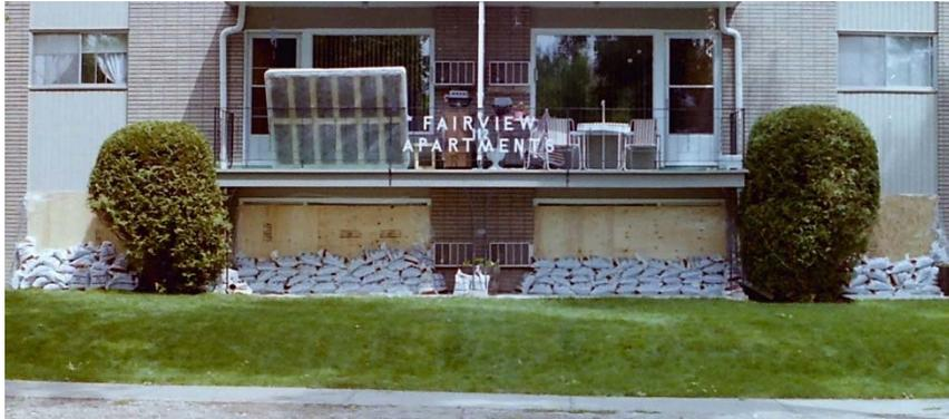
**Figure 8.1** Example of simple flood proofing measures: blocking low openings with plywood and sandbags. (Photo by F. Hicks.)
