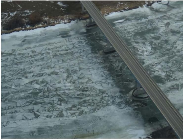
**Figure 8.5** Ice surface appearance after completing of ice cutting on the Red River, Manitoba. Note the triangle-like shapes visible on the ice surface where the cutting occurred. *(Photo courtesy of S. Clark.)*
