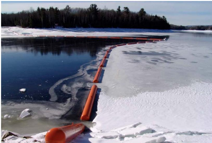
**Figure 8.11** Example of ice cover forming upstream of an ice boom.
