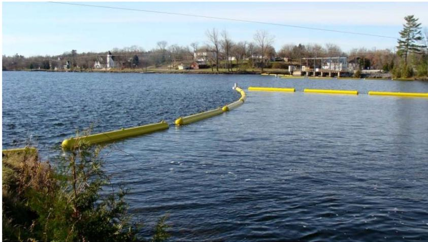
**Figure 8.10** Example of an ice boom in place prior to freeze-up.
