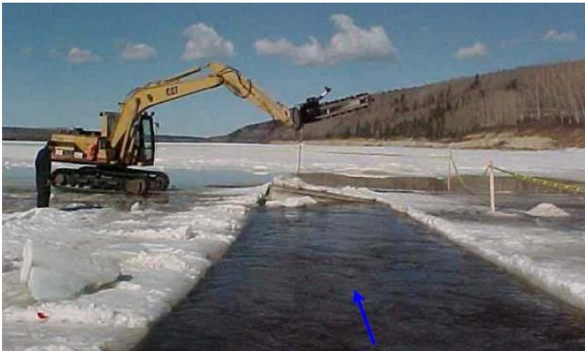
**Figure 8.8** Ice saw being used to cut up an ice bridge on the Athabasca River, Alberta. (Photo courtesy of Alberta Environment and Sustainable Resource Development.)
