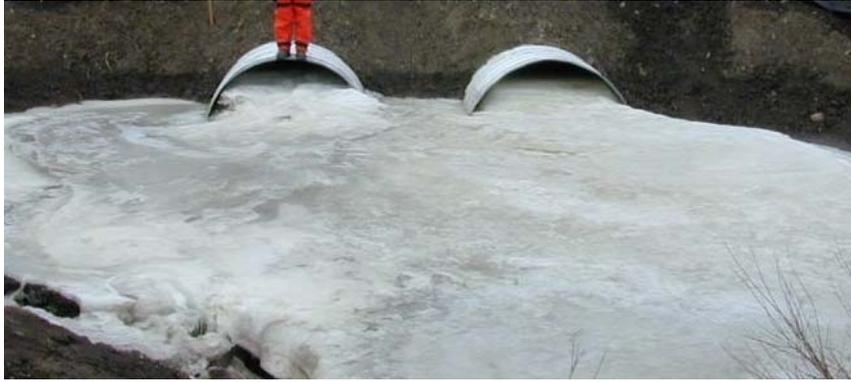
**Figure 2.37** Example of culvert icing. (Photo by F. Hicks.)
