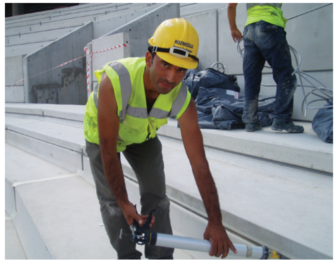
MasterSeal joint sealants were used in the Besiktas football stadium, Istanbul
