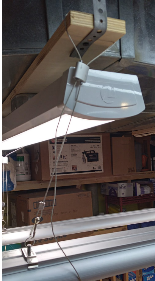
Figure 7: Mounting of Grow Lights
