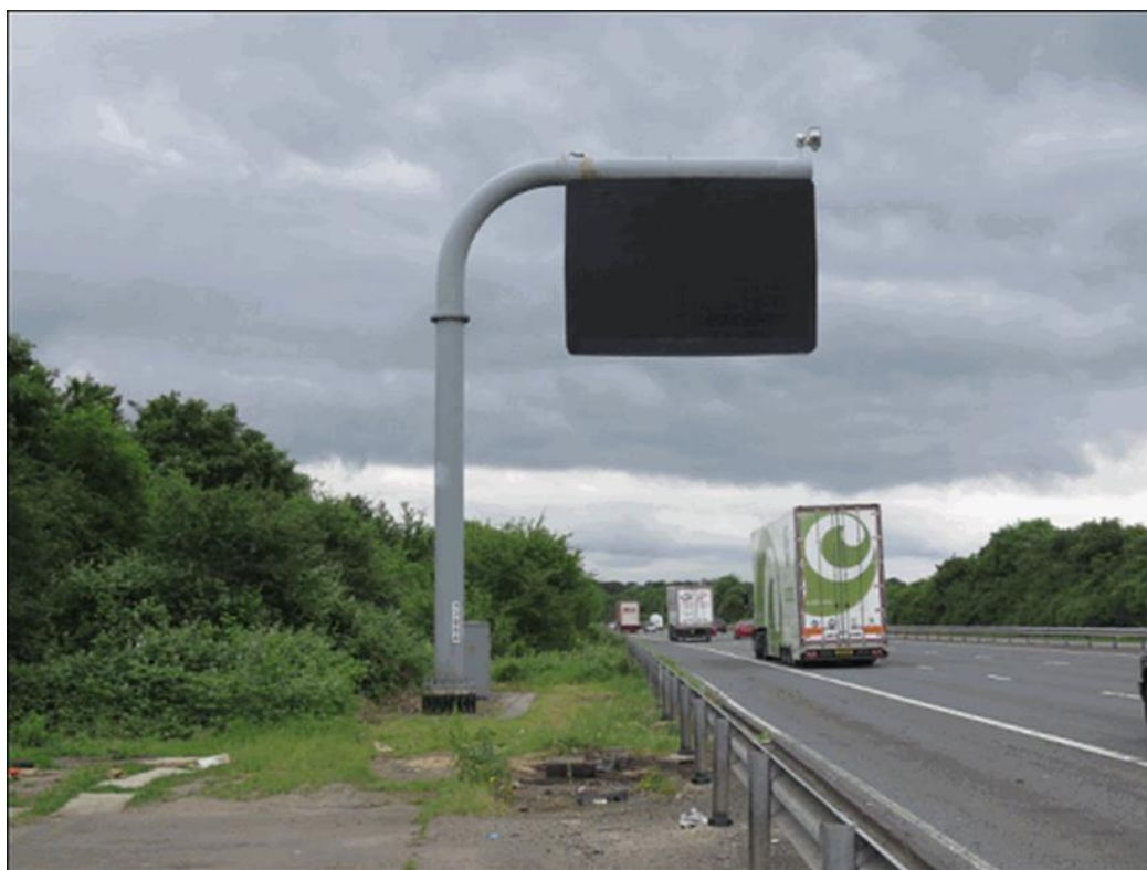
Figure 3-12 View of MS4 Cantilever Gantry 12 Looking South
