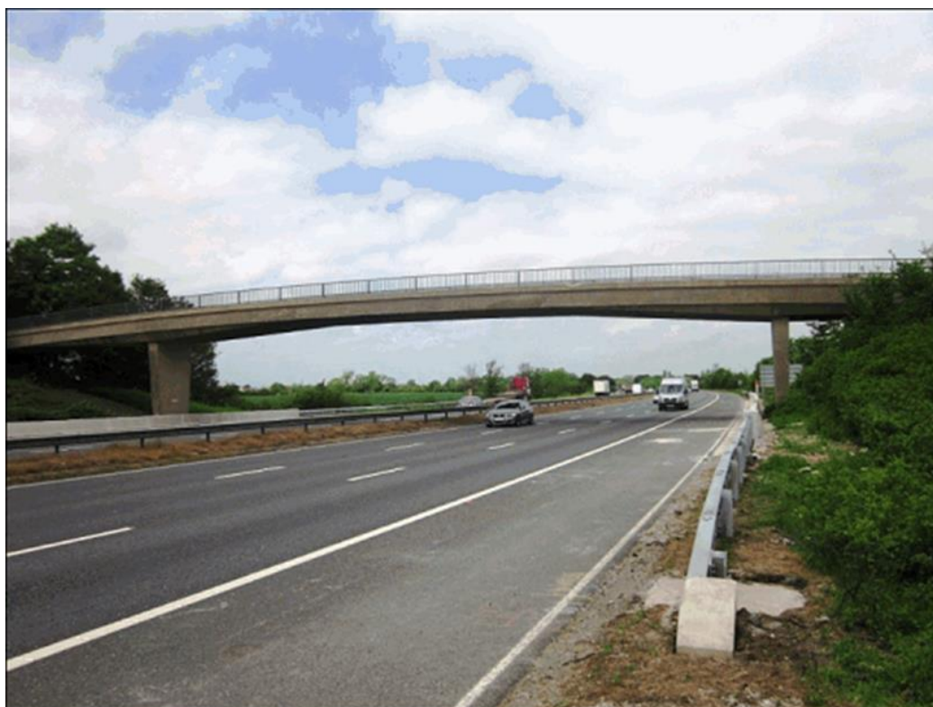
Figure 3-1 South Elevation of Green Farm Access Bridge
