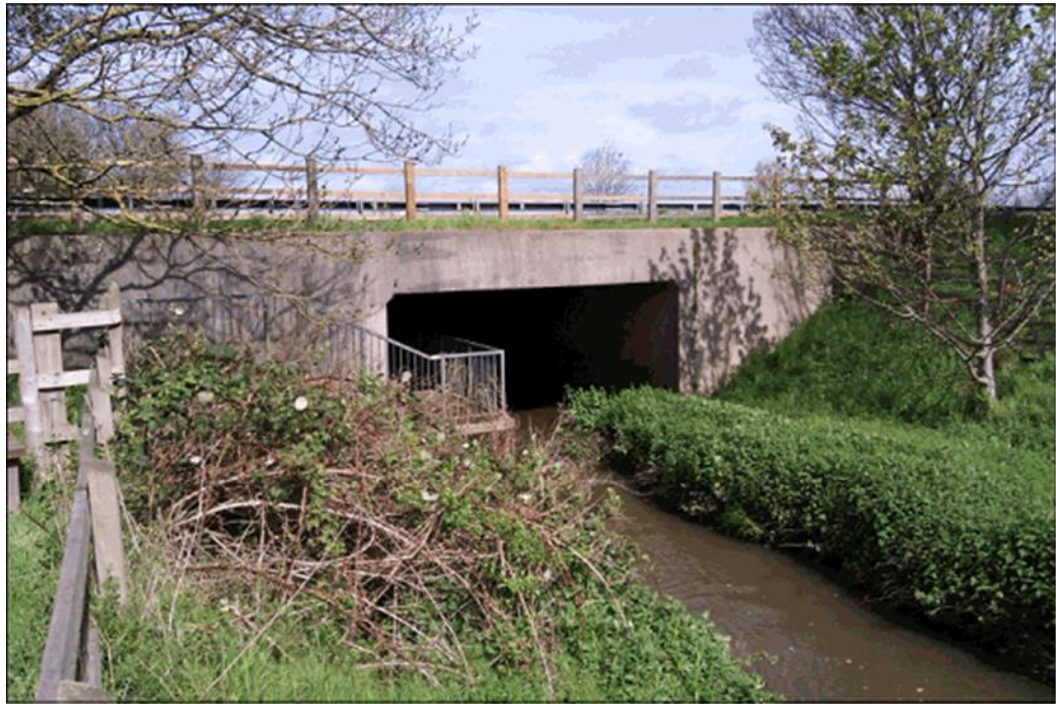
Figure 3-8 East Elevation of River Celt Culvert
