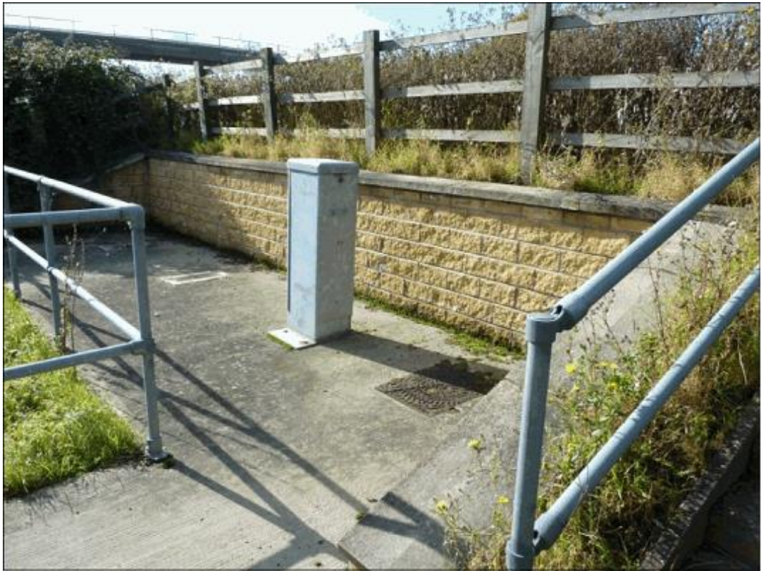
Figure 3-10 Typical Arrangement of a Comcab Retaining Wall
