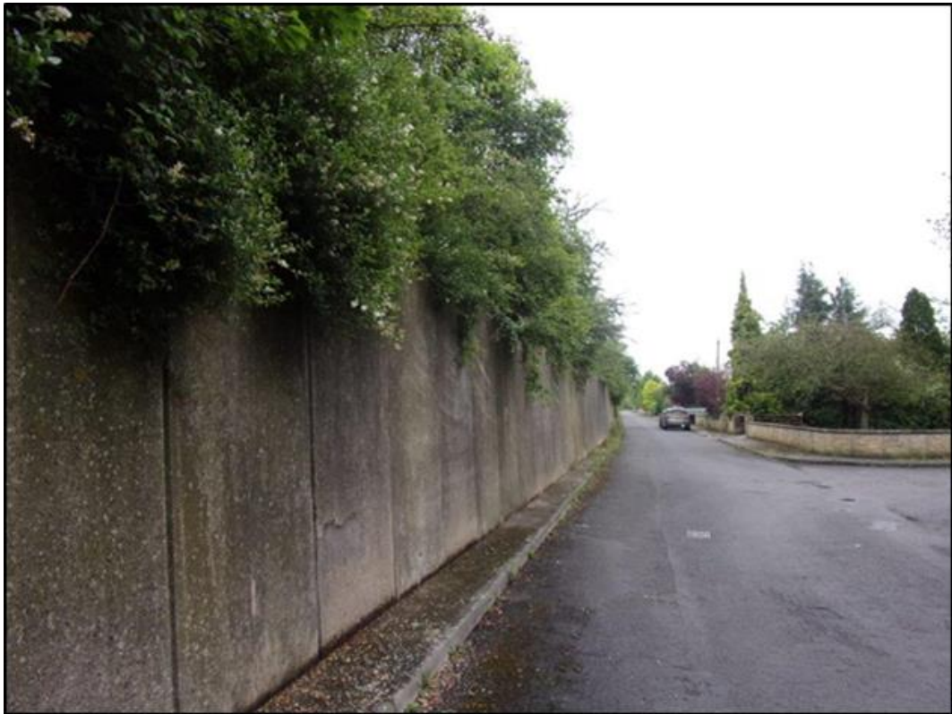
Figure 3-5 View East along Withybridge Gardens Retaining Wall
