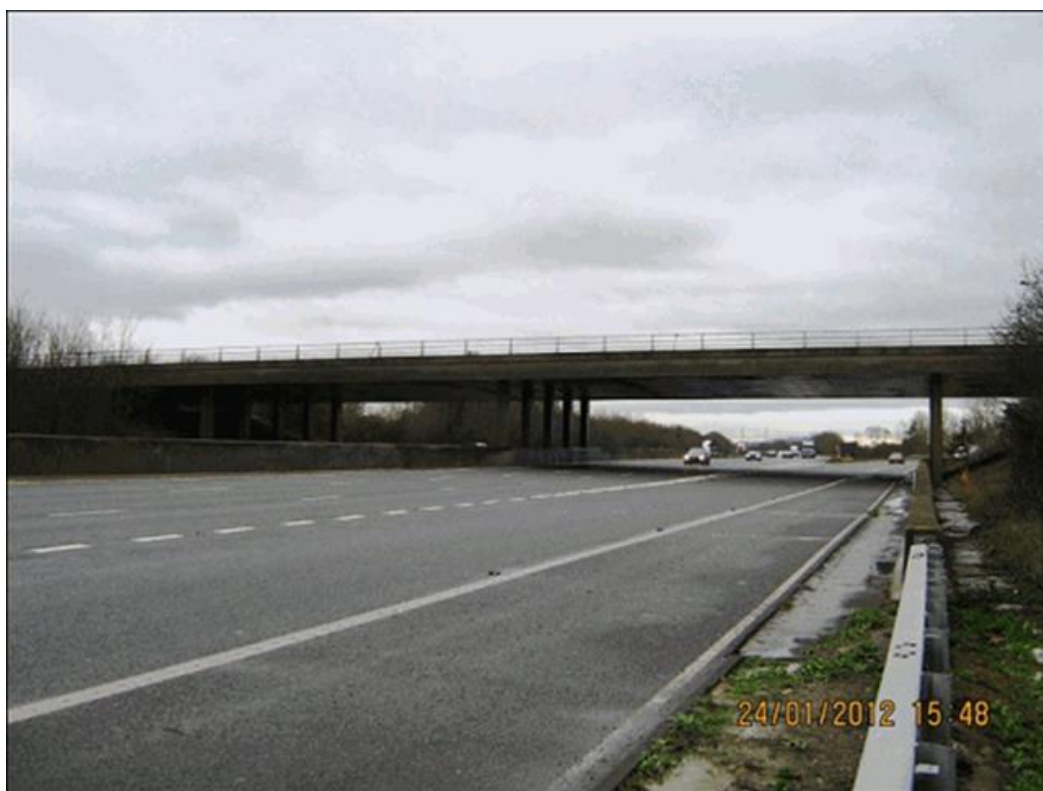
Figure 3-4 North Elevation of Piffs Elm Interchange Bridge
