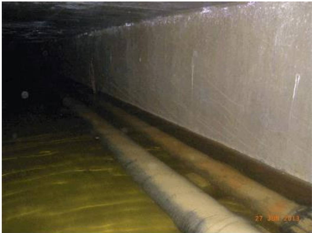
Figure 3-6 Typical View inside Piffs Elm Service Culvert
