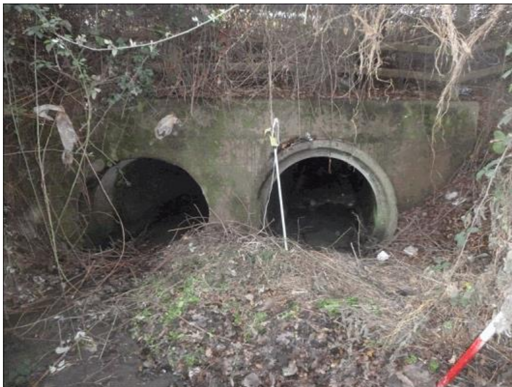
Figure 3-3 East Elevation of Barn Farm Culvert
