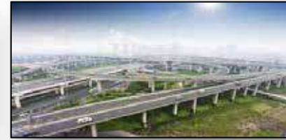
Transportation: Highways and Bridges
