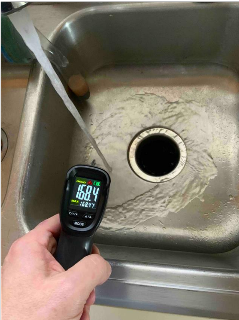
7.2 Item 1(Picture) Hot water temperature
