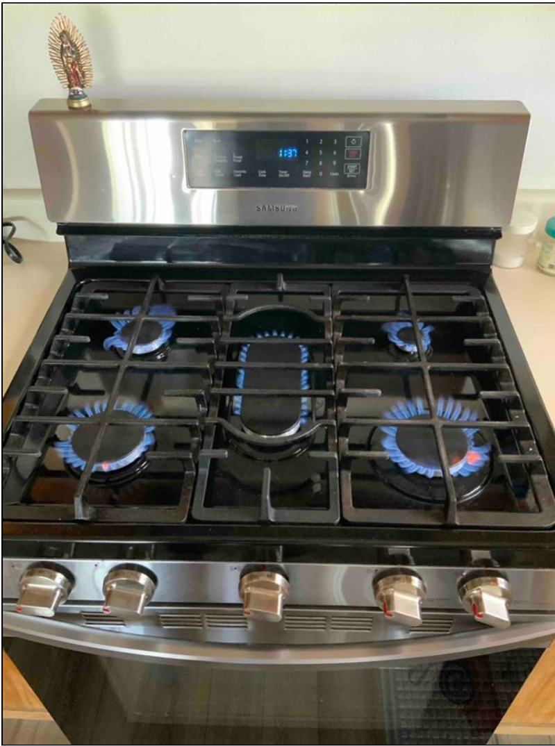
4.1 Item 1(Picture) Stove top operating
