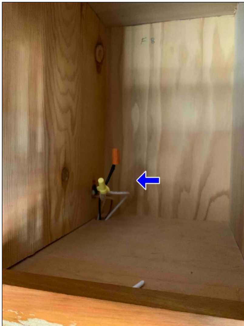
1.4 Item 1(Picture) wire splices in the kitchen cabinet above the stove fan
