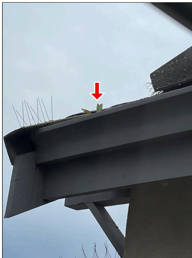
2.4 Item 1(Picture) debris in gutters
