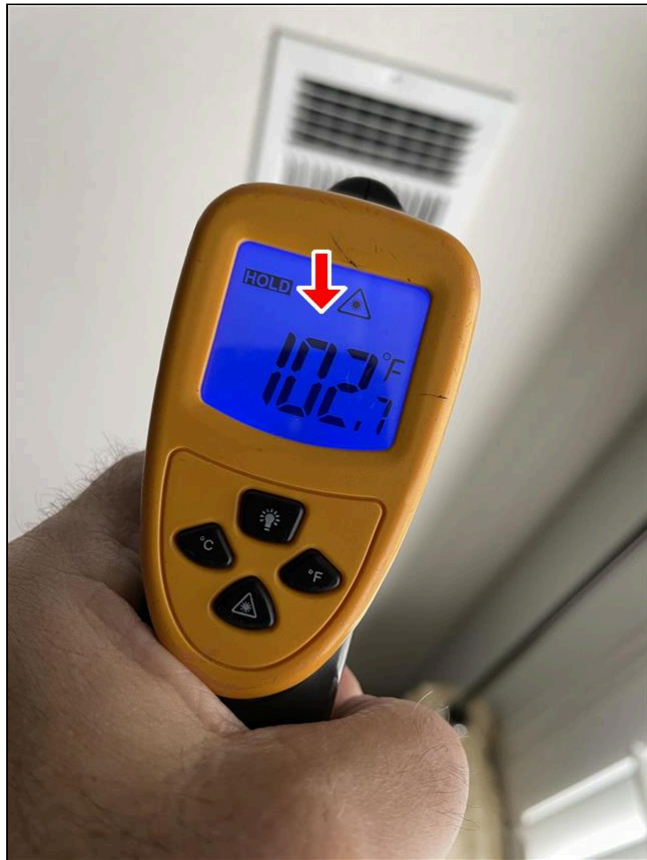
8.4 Item 1(Picture) furnace operational
