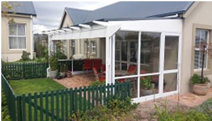
Photo 7 – Unit 20 - Short side of patio enclosed with sliding door
