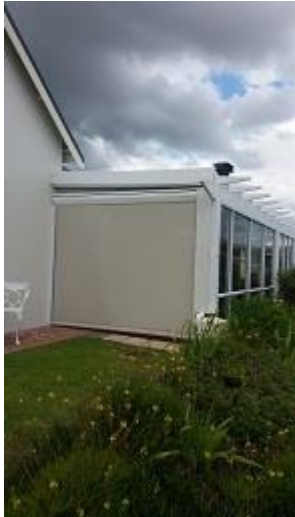
Photo 6 – Unit 69 – Patio enclosed 2 of 3 sides
