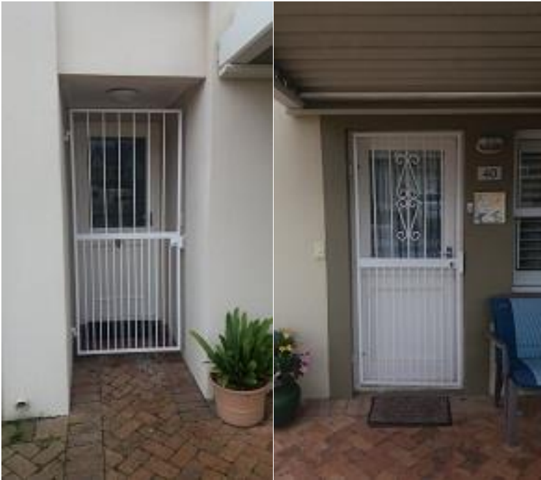
Photo 21 & 22 - Examples Security Gates (trellis doors only permitted on the inside)
