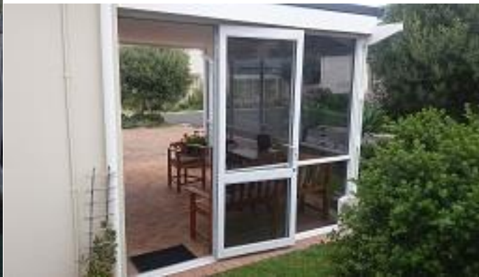
Photo 8 – Unit 21 – 2 of 3 sides enclosed with door
