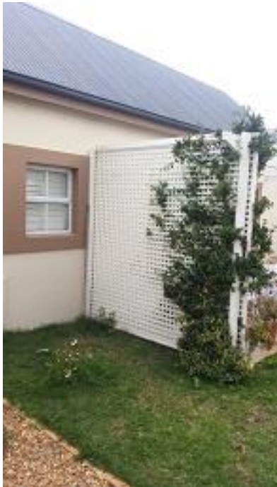
Photo 14 & 15 – Unit 87 – Patio enclosed on 1 side (short side) with white timber lattice screen
