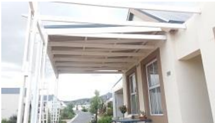
Photo 12 – Unit 83 – Corrugated roof covering over pergola on patio
