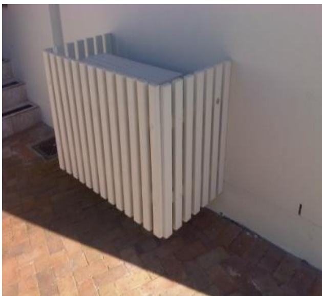
Photo 28 – Air conditioner enclosure
