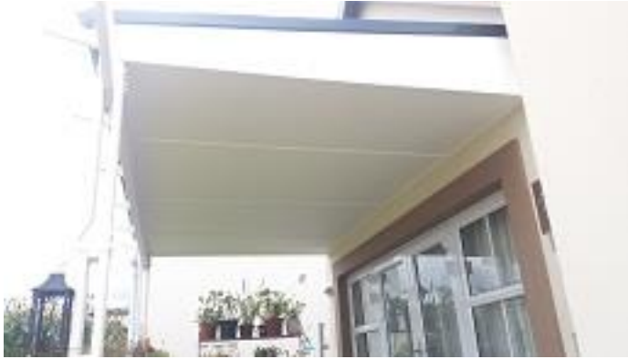
Photo 13 – Unit 3 Pergola covered with corrugated roof sheets and ceiling added
