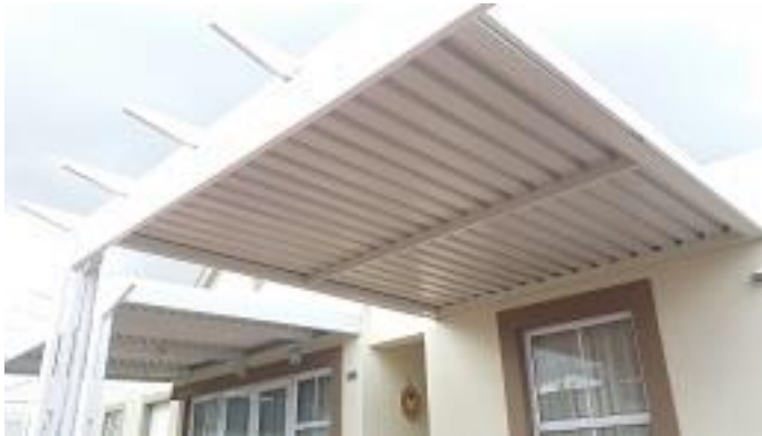
Photo 11 – Unit 94 Pergola on patio covered with white aluminium louvre
