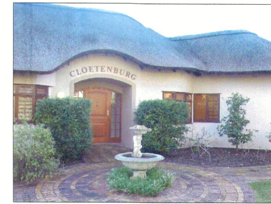
EXIST FRONT DOOR
