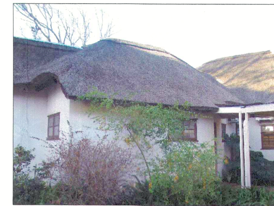
VIEW OF AREA TO BE ADDED ON TO
